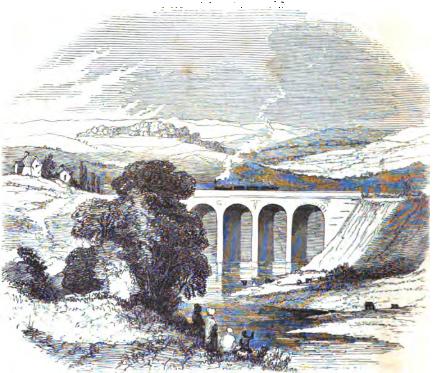
DRYFE SANDS VIADUCT.
